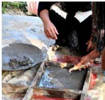
Everything was made locally, the square paves were made combining local knowledge and advanced knowledge of the use of a wired mesh to make it stronger for heavy use by children
