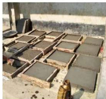
Everything was made locally, the square paves were made combining local knowledge and advanced knowledge of the use of a wired mesh to make it stronger for heavy use by children
