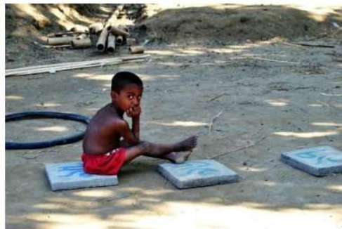
Everything was made locally, the square paves were made combining local knowledge and advanced knowledge of the use of a wired mesh to make it stronger for heavy use by children
